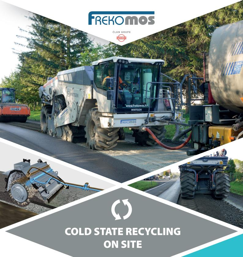
Cold state recycling on site technology is based on the secondary use of materials already built into the construction of the road surface without heating. Process involves milling and granulating damaged asphalt layers which are then rebound, placed again and compacted.
